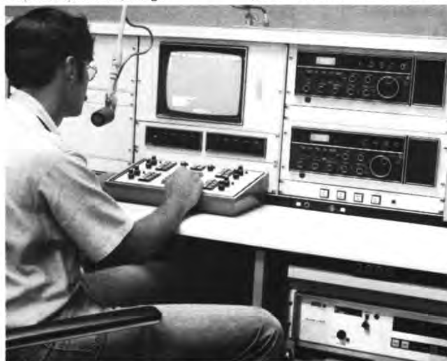
Screens at each operator's console display a variety of information including transmitter, frequency, antenna, power and mode.
